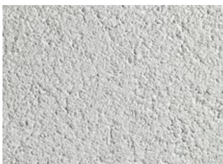
Hladená technika | Smoothing technique
