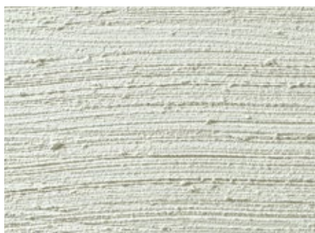
Metličkovanie | Broom technique
